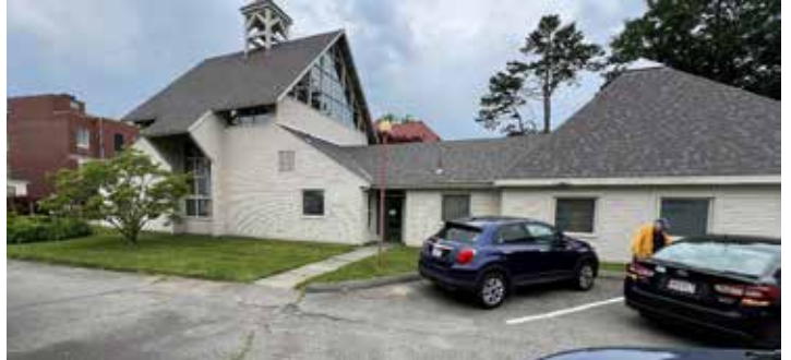
The Exterior, Showing the Side Entrance, which has just been upgraded with a new walkway and sturdy railing. Note the High A-frame style roof filled with glass panels
